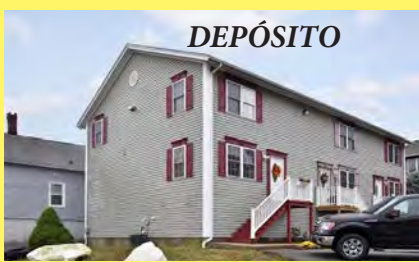
CENTRAL FALLS Condomínio $229.900
